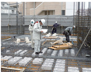
Housing performance evaluation (Reinforcement arrangement inspection)
