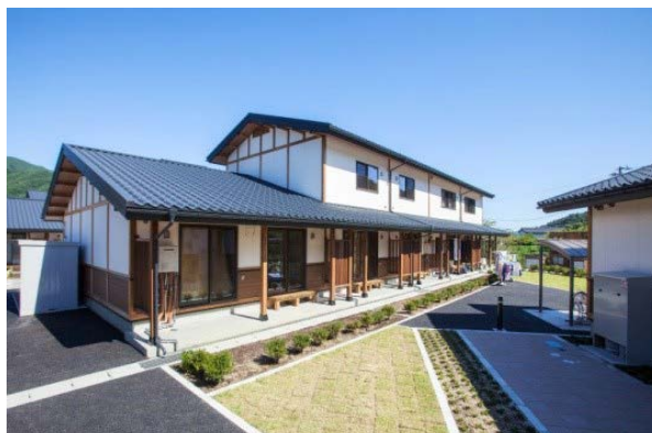
Photo 3-2-5: Example of Public Housing Provided for Disaster Relief (Otsuchi-cho, Iwate Pref.)
