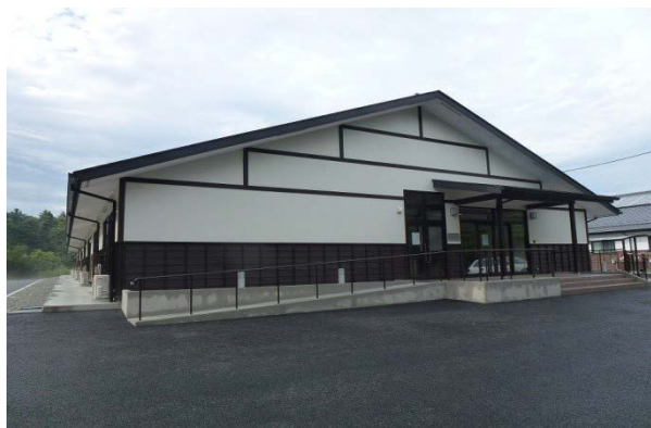
Photo 3-2-4: Example of Public Housing Provided for Disaster Relief (Soma City, Fukushima Pref.)
