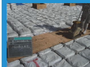
⑨土間部土間転圧
