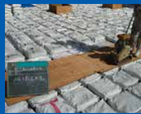
⑨土間部土間転圧
