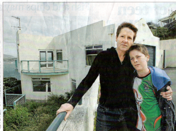
No home sweet home: Miranda Patrick and son Cameron Simpson, 11, outside their leaky and unoccupied house, which overlooks Wellington Heads. Photo PHIL REDD
