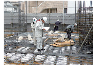
Housing performance evaluation (Reinforcement arrangement inspection)
