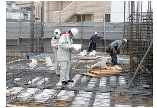
Housing performance evaluation (Reinforcement arrangement inspection)
