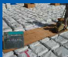
⑨土間部土間転圧
